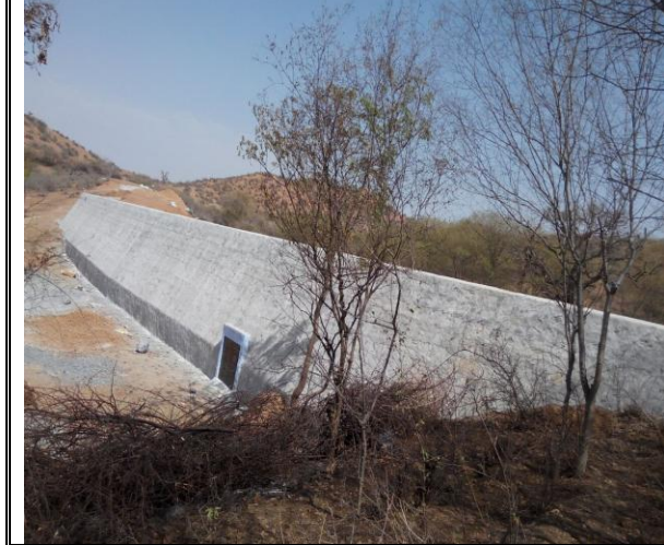
2016: the Uprala Wala Dam, Dist. Sikar, Rajasthan, India
