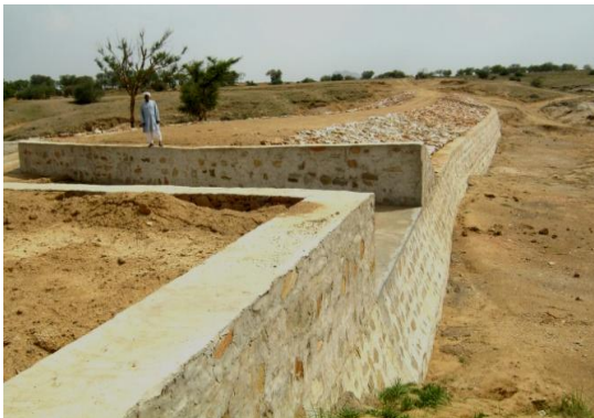
2014: the Moutala Wala Dam, Dist. Sikar, Rajasthan, India
